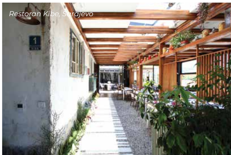
Restoran Kibe, Sarajevo
